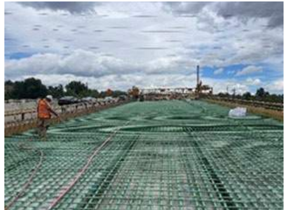
Figure 13. Tied reinforcement for the eastbound Fountain Creek Bridge deck.
