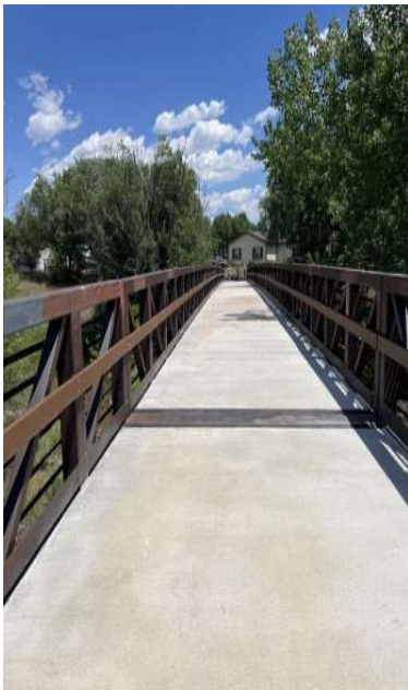
Figure 42. Templeton Gap Bridge Redecking. Complete Spring 2024.
