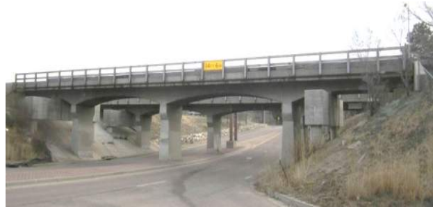
Figure 27. Existing Fontanero Bridges.
