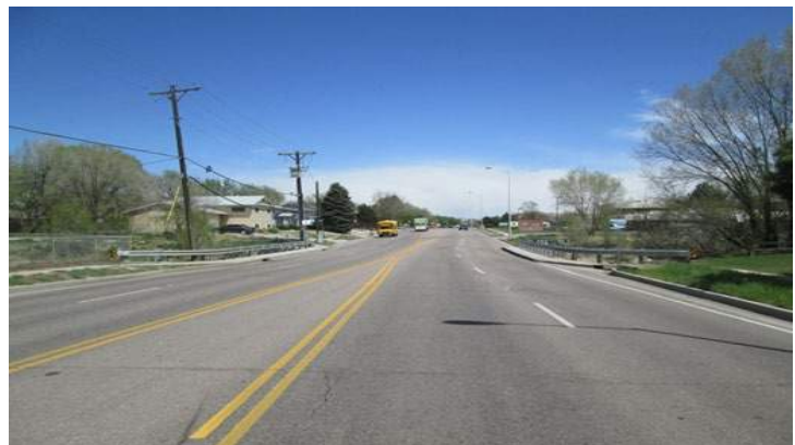
Figure 17. Narrow roadway over existing Galley Road Bridge.
