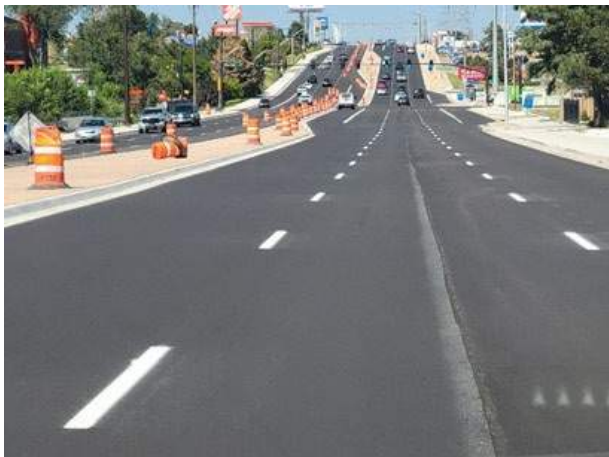
Figure 6. Completed paving and striping.
