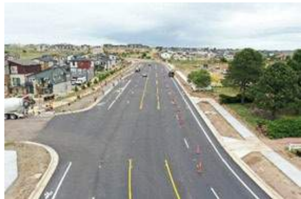
Figure 25. Tutt Blvd. open to traffic 8/26/2024.
