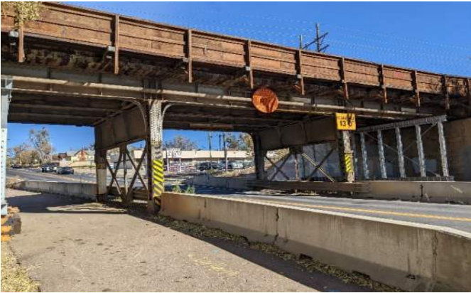
Figure 28. View of RR Bridge from NB Tejon Street.
