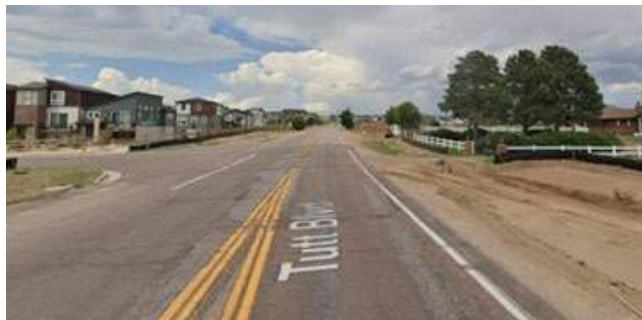
Figure 24. Tutt Blvd. Before Construction.
