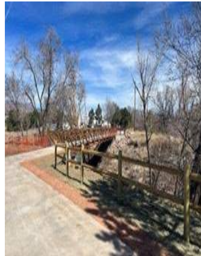
Figure 43. Construction complete for Mesa Creek Confluence Pedestrian Bridge.
