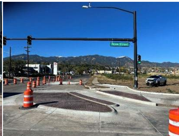
Figure 19. Bike lane channelizing island and new concrete pavement panels.
