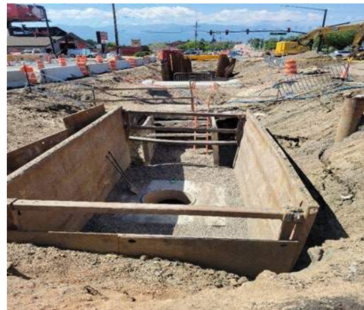
Figure 7. Manhole for 42” sewer.
