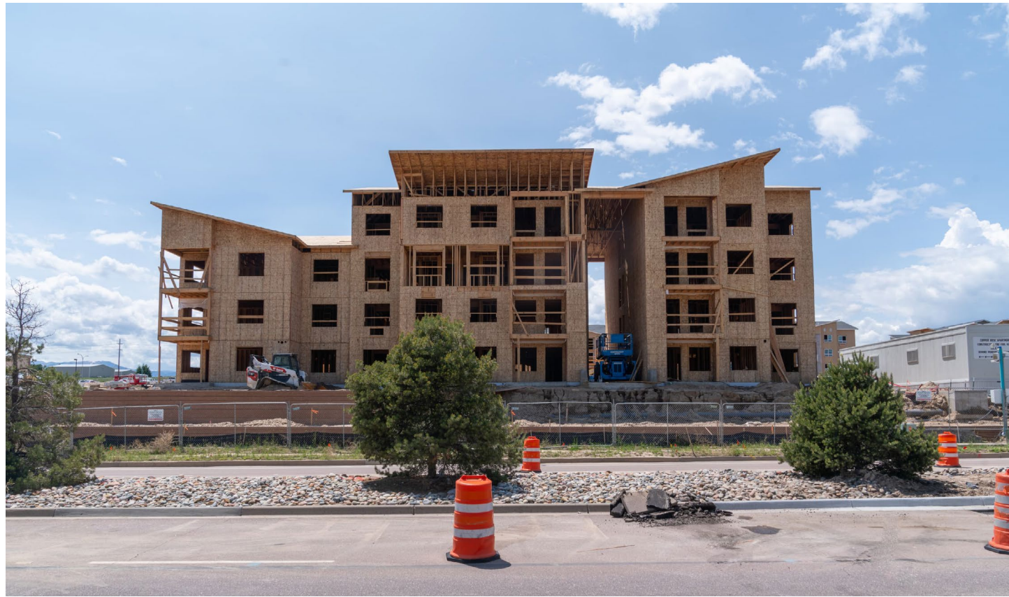
Multi-family development construction
