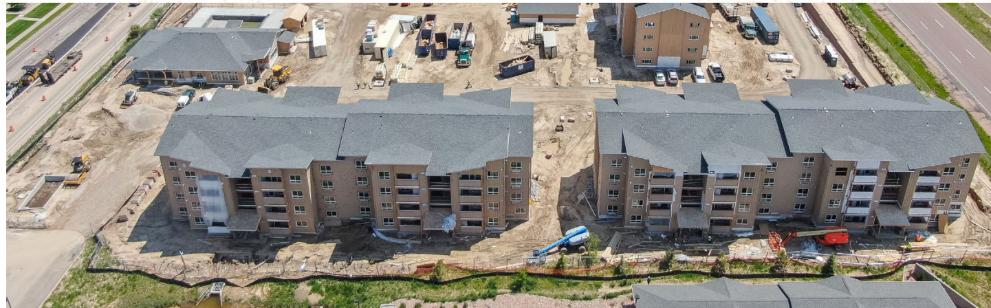
Multi-family under construction on Woodmen Rd
