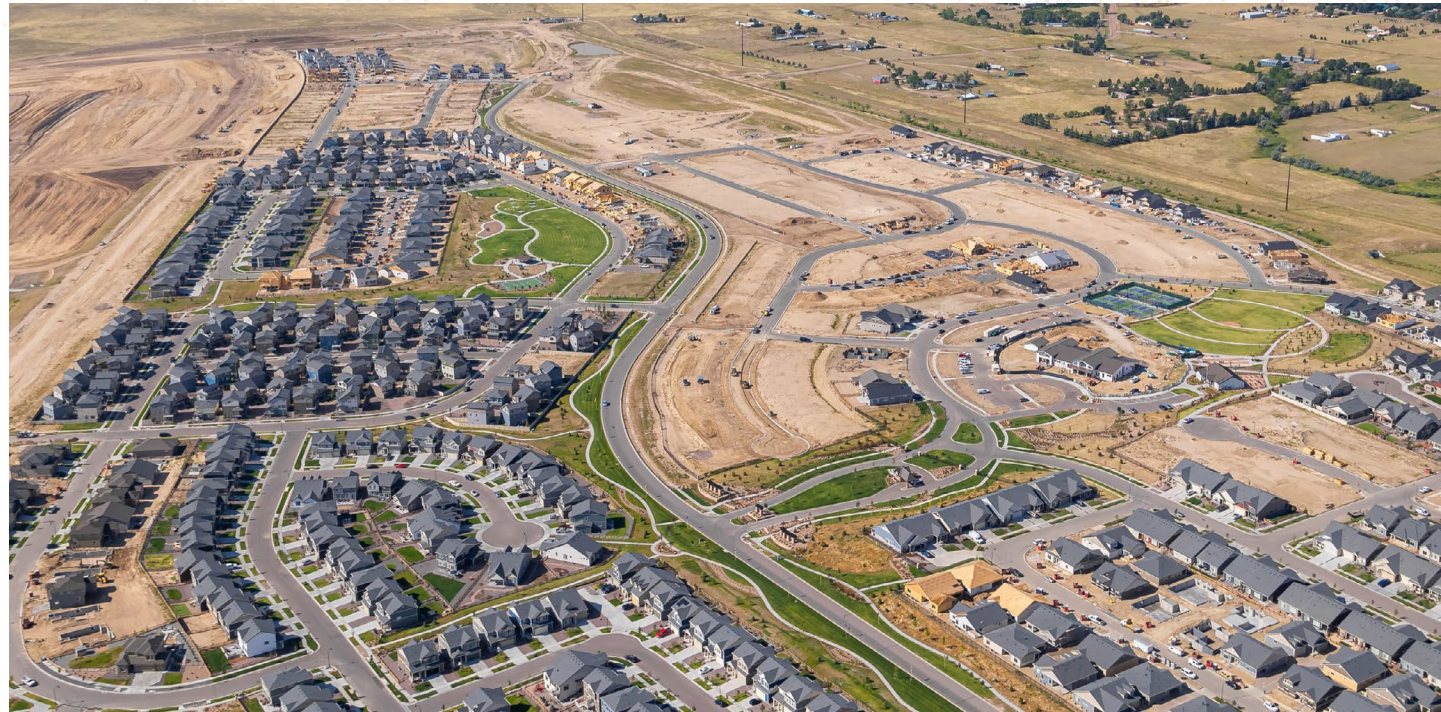
Banning Lewis Ranch development and construction
