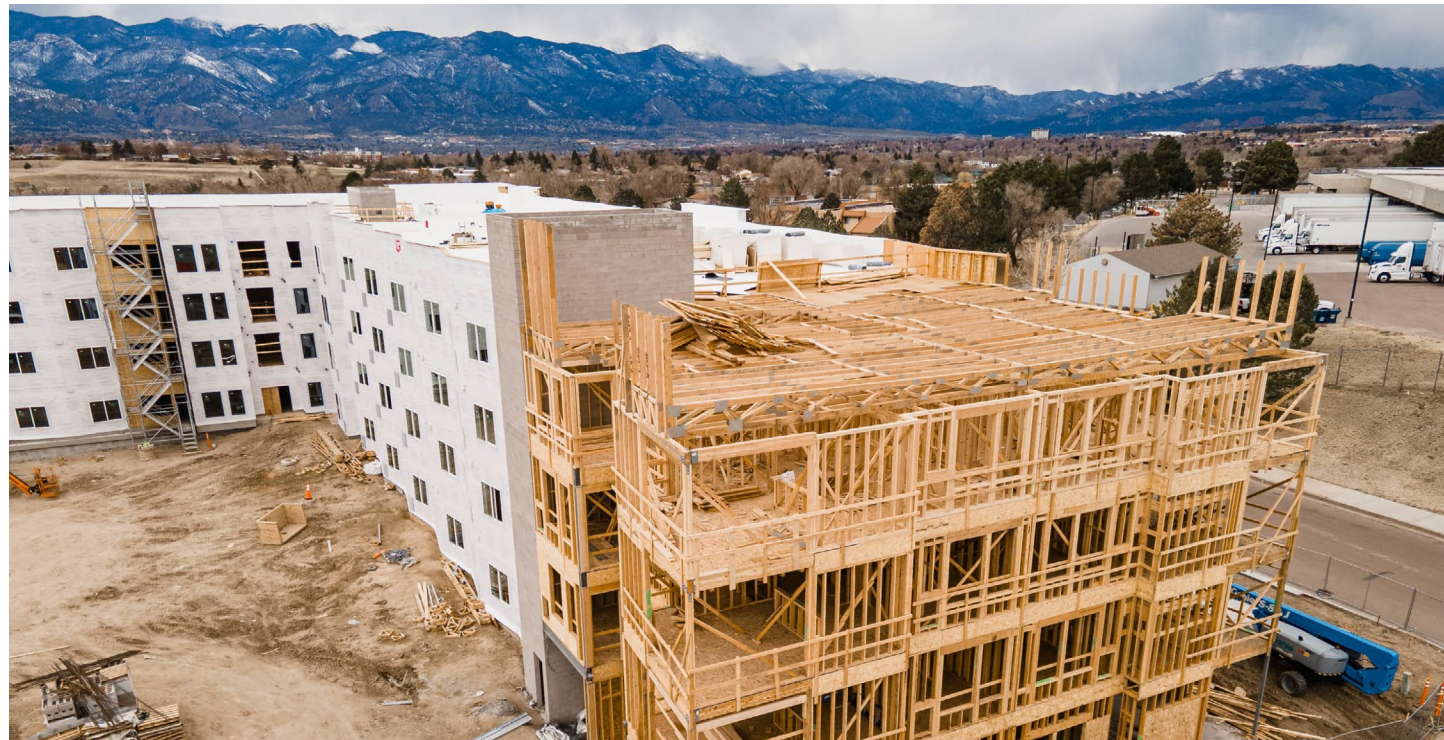
Affordable housing development under construction
