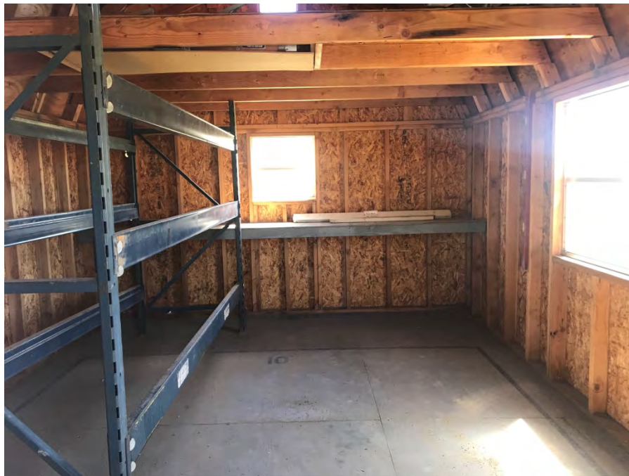
Photograph 12: View inside empty shed.
