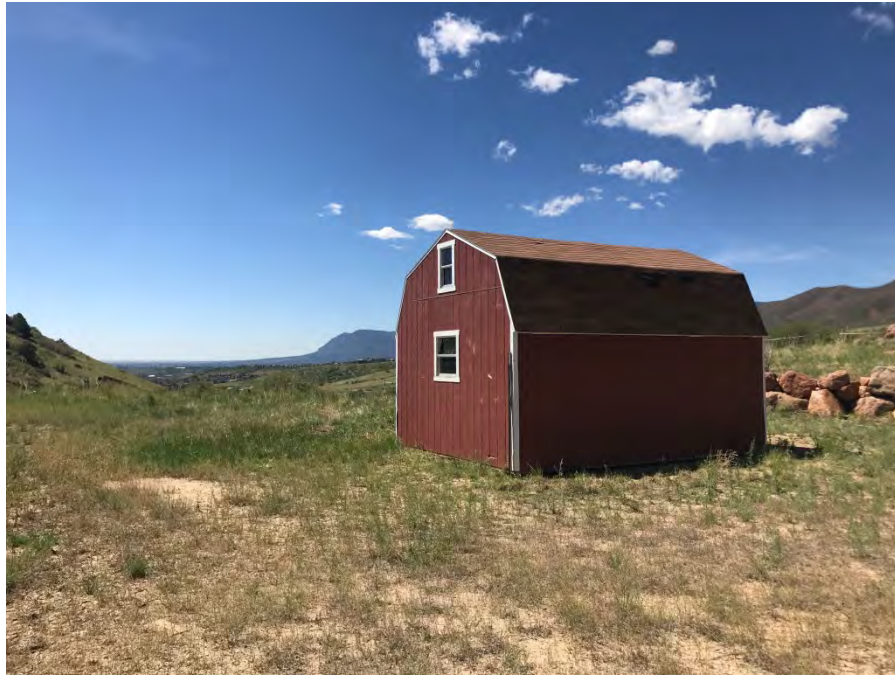
Photograph 11: View of empty shed located on the southeast corner of the site.
