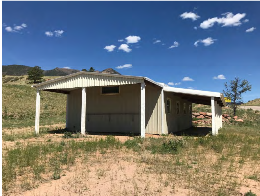
Photograph 9: View of empty structure located near the eastern boundary of the site.
