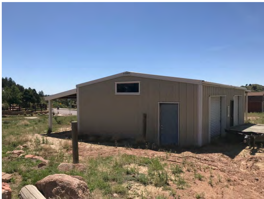
Photograph 8: View of empty structure located near the eastern boundary of the site.
